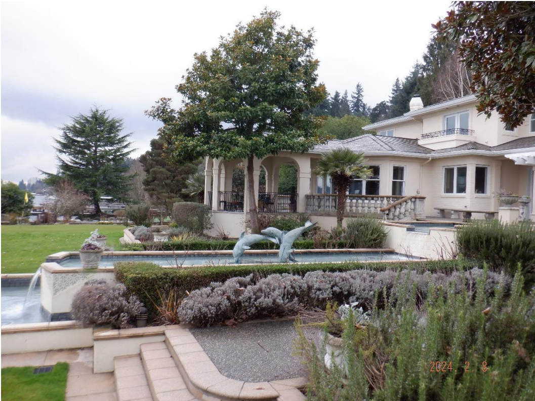
Looking south across back of house
